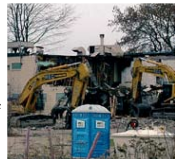
The old paint factory is demolished!!
